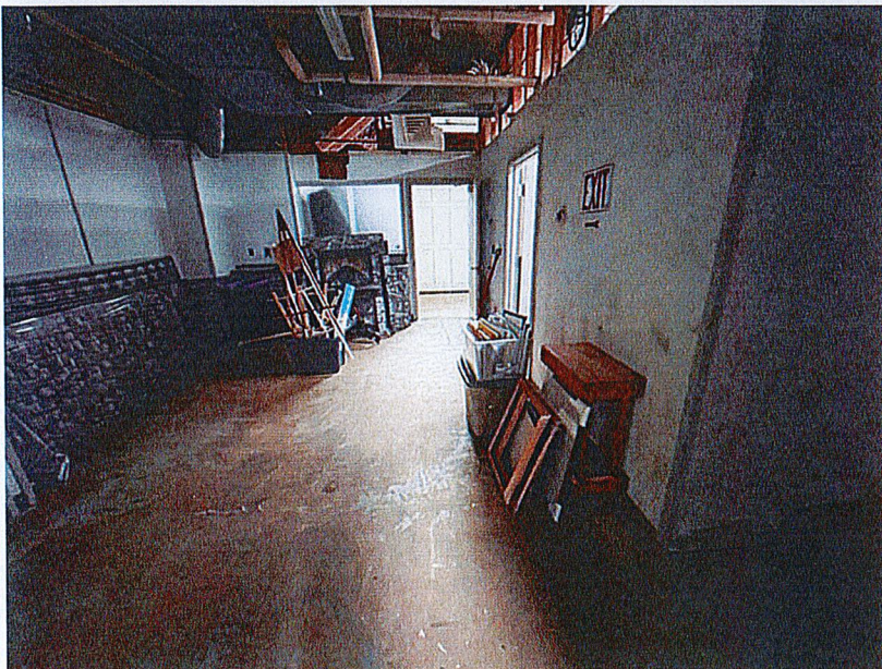
GRADE LEVEL AREA FOR ADA ELEVATOR
