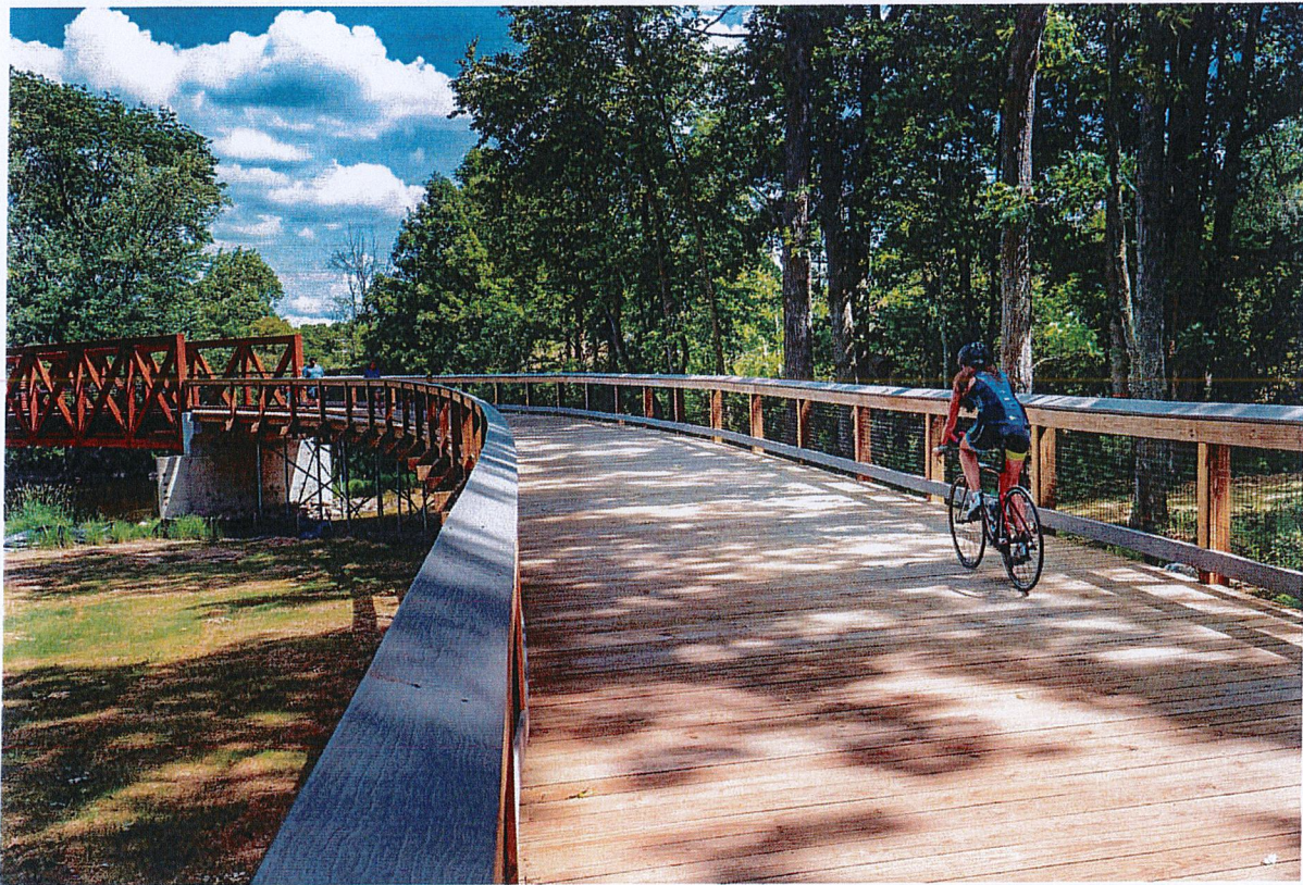
A new segment of the B2B Trail off Huron River Drive in Dexter.
